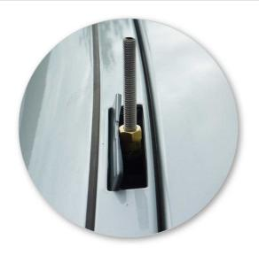
Close all fixed-point covers so they rest on the grubscrew and place pads over grubscrews.
